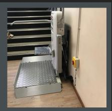
We have installed a V6R lift at a University in Cape Town. A V6R lift is economical and is a space saving platform stair lift providing a popular and versatile access solution for wheelchair users. The wheelchair user rolls onto the platform, safety bars lower, and a constant pressure joystick, operated by the wheelchair user, controls movement along the staircase. A perfect addition to a University.
